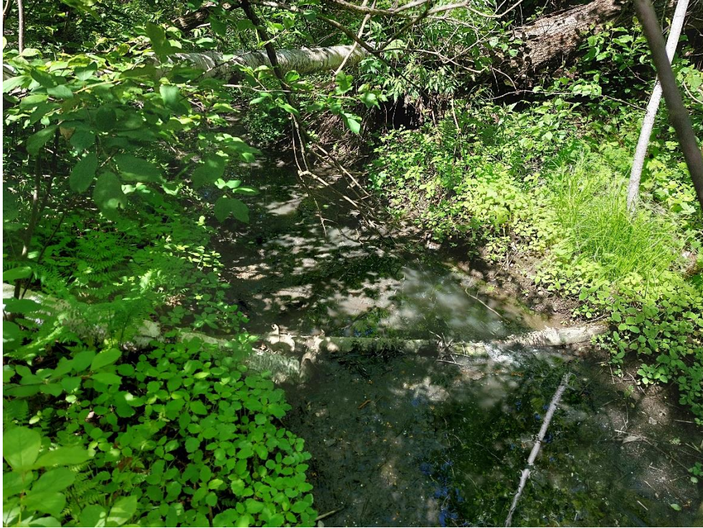
Photo 5: View of sludge in drainage channel (May 31, 2022)
