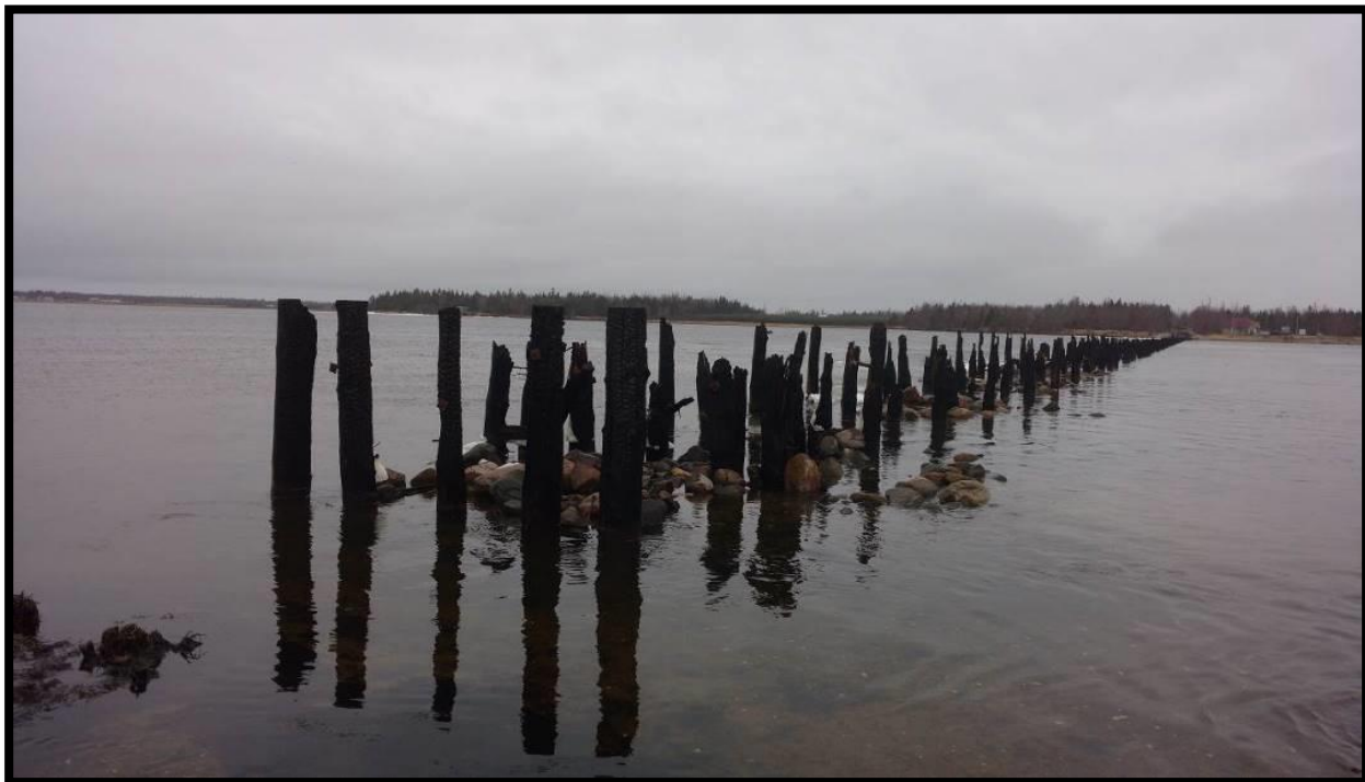
Photo No. 1: Inkerman Bridge (2018)
