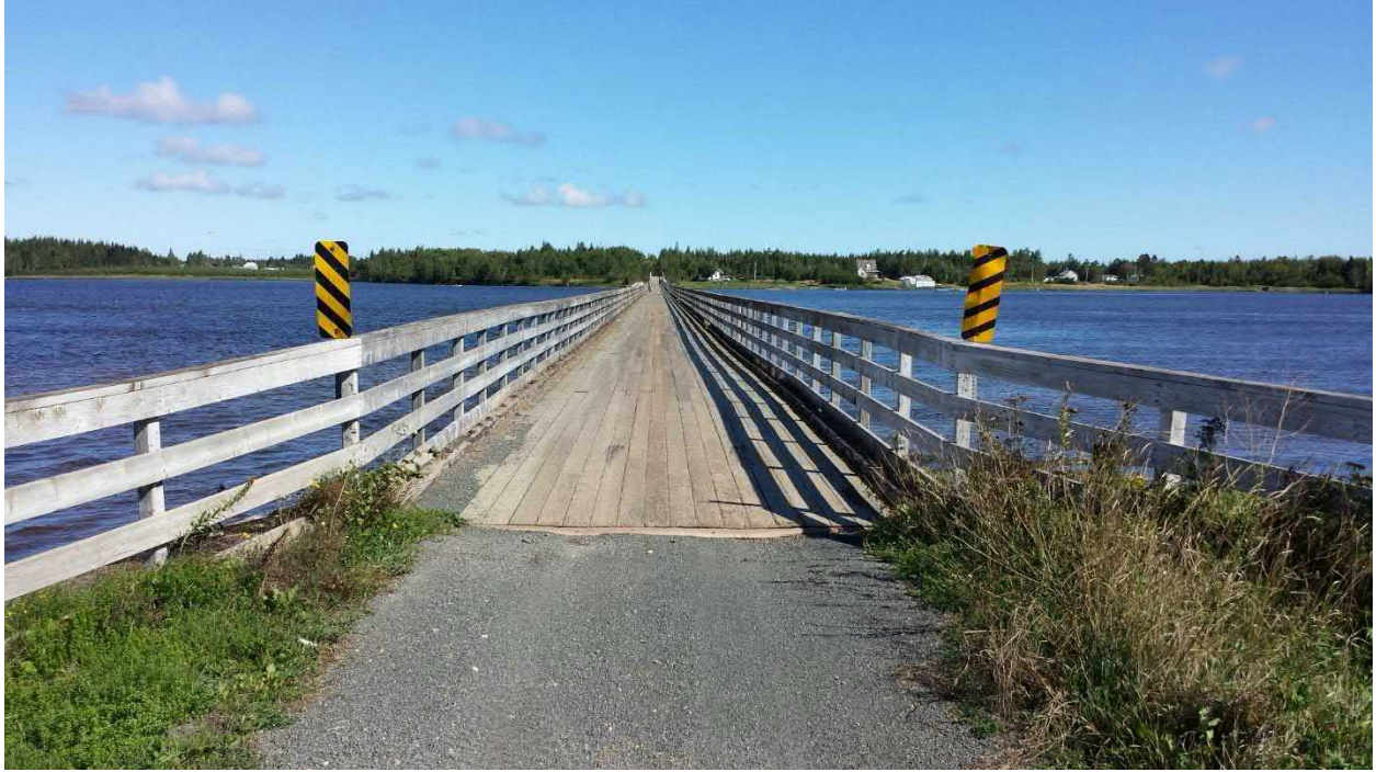
Photo No. 1: Inkerman Bridge Pre-Fire Looking North (2016)
