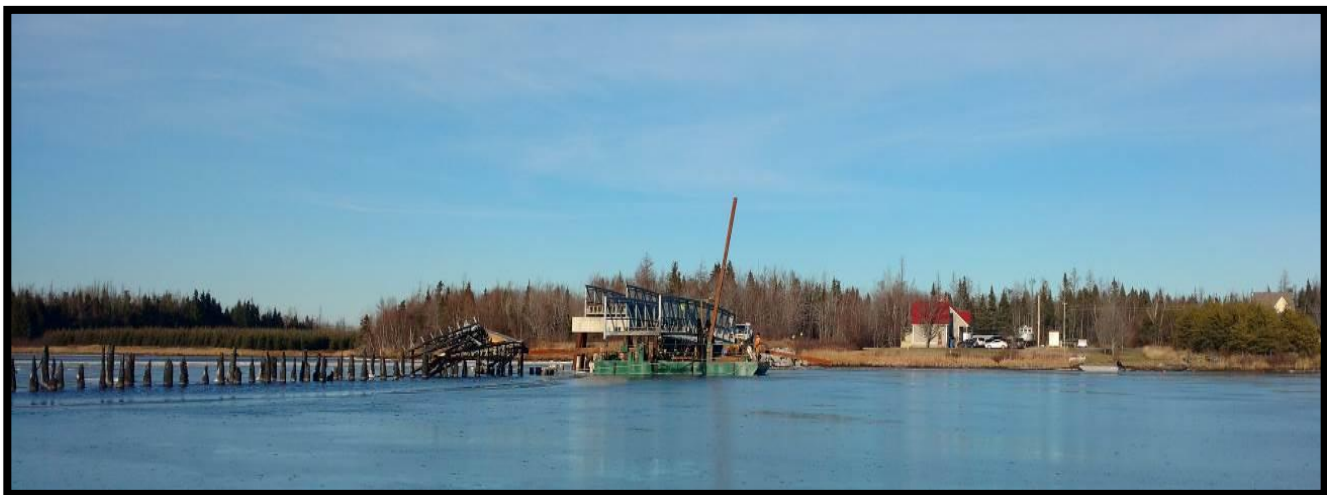
Photo No. 3: Remnants of Bridge and Northeastern Approach (Looking North, November 30, 2017)
