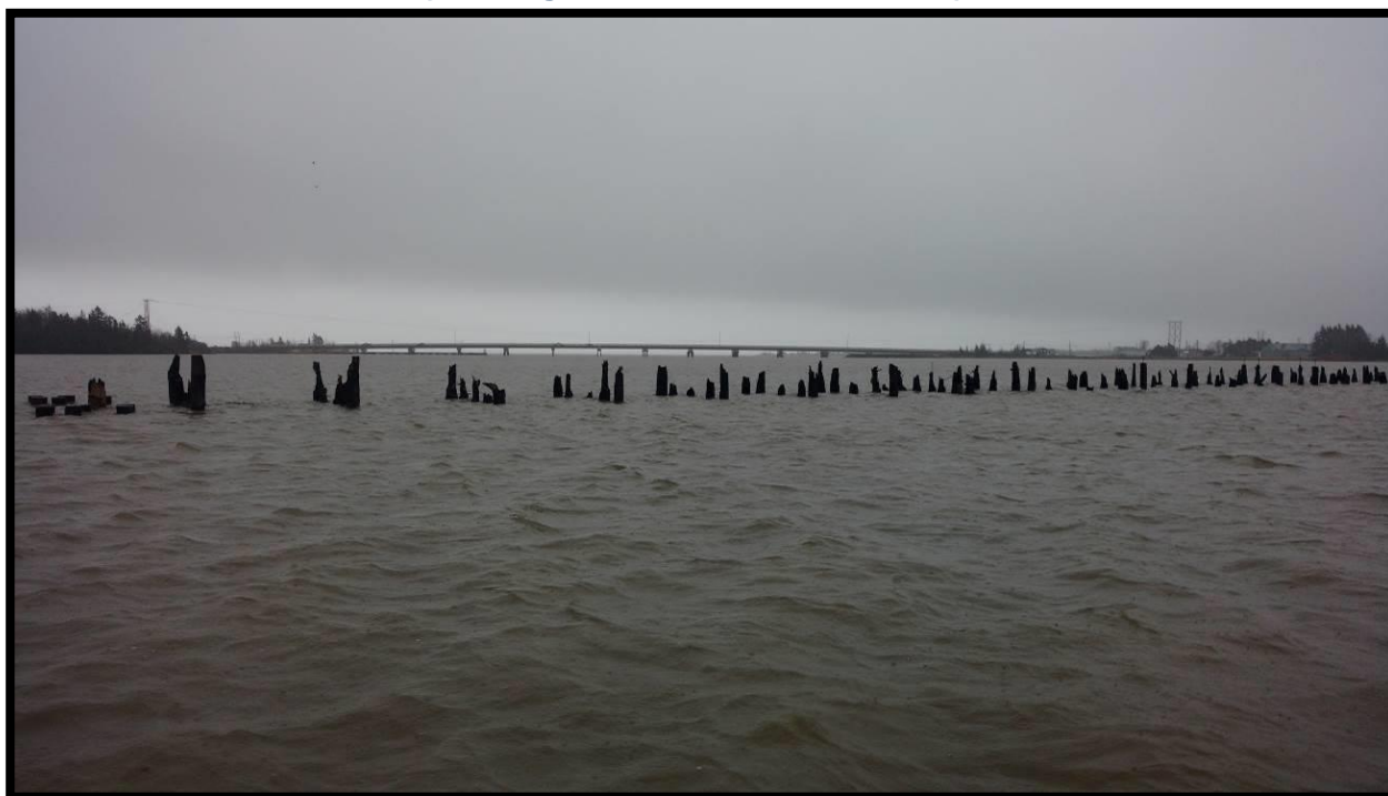
Photo No. 4: Charred Creosote-treated Wooden Piles (Looking South, December 6, 2017)
