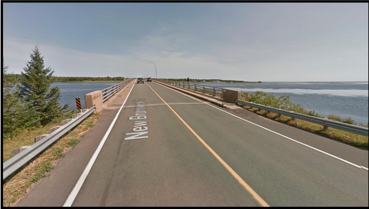
Photo No. 2: Route 113 Bridge (GoogleEarth©)
