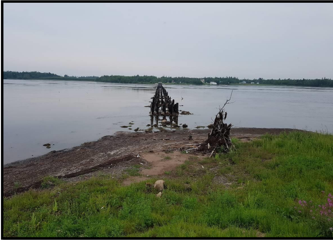
Photo No. 6: Southwestern Approach
