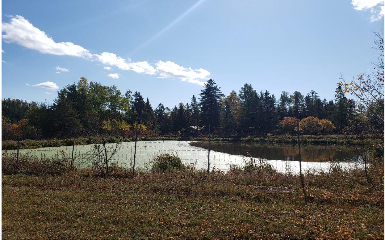
Photo 1 - Looking southeast at the Everett Lane Lagoon (October 2020).
