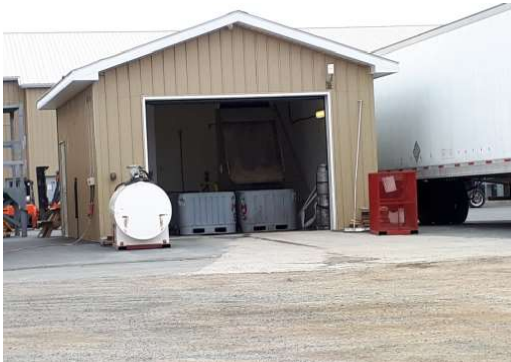
Photo No. 17: Solids Removal Building and Portable 1120 L Fuel Oil Tank
