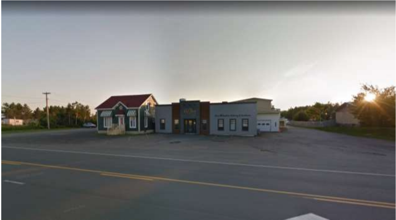
Photo No. 1: Existing McGraw Seafood Inc. Plant, 3113 Rue Principale (GoogleMaps©)
