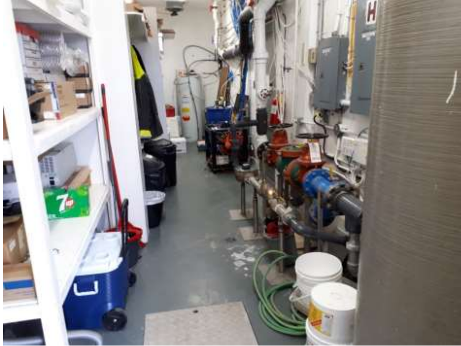
Photo No. 3: Production Well No. 2 (PW2) (foreground)
