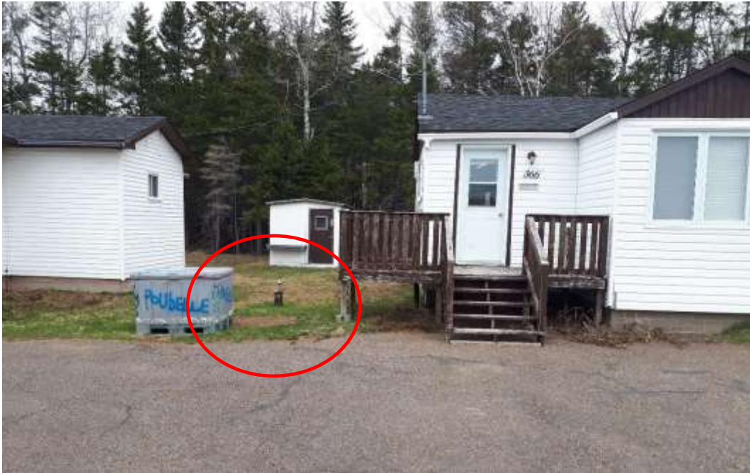
Photo No. 7: Cottage Domestic Well (Well ID 0007575) (Circled in Red)
