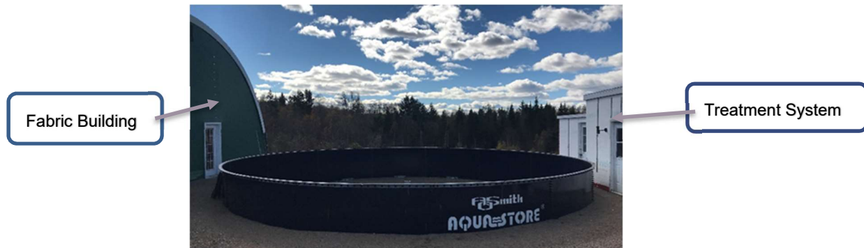
Figure 5 Existing Steel Tank (Rear of JLH Building)
