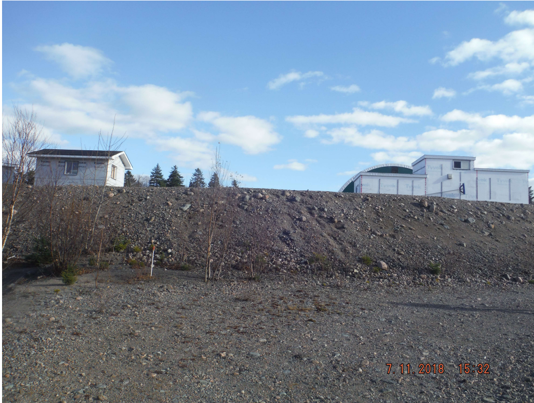
Photo 5 Looking to Rear of Existing Hatchery Showing Amount of Fill Material
