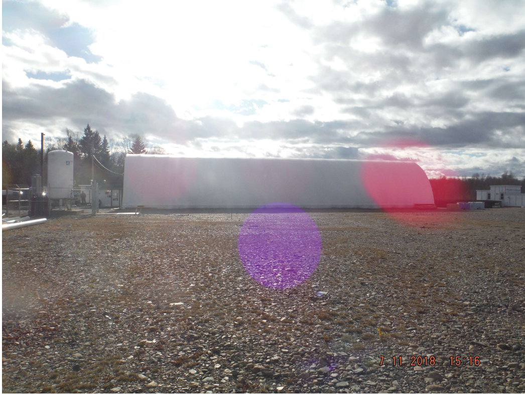
Photo 3 Side View of Existing Hatchery Looking Southwest
