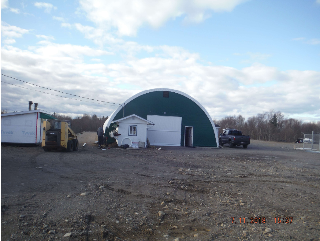
Photo 7 Looking to Front of Existing Hatchery
