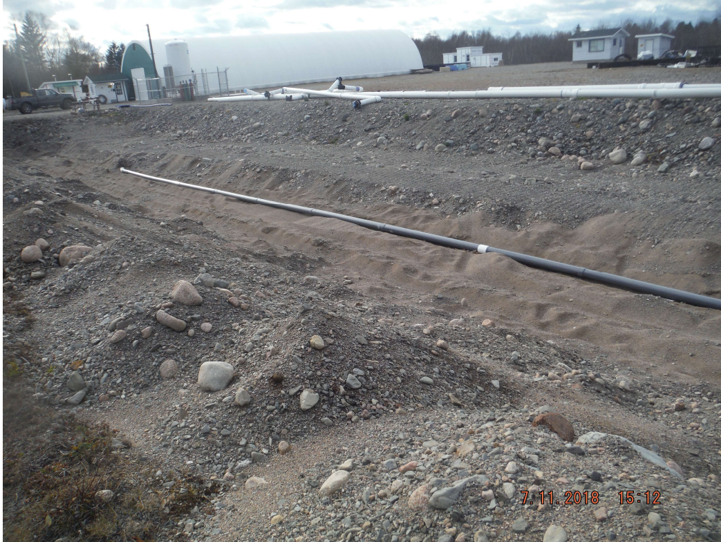
Photo 1 Approximate Location of New Building (Existing Hatchery in background)
