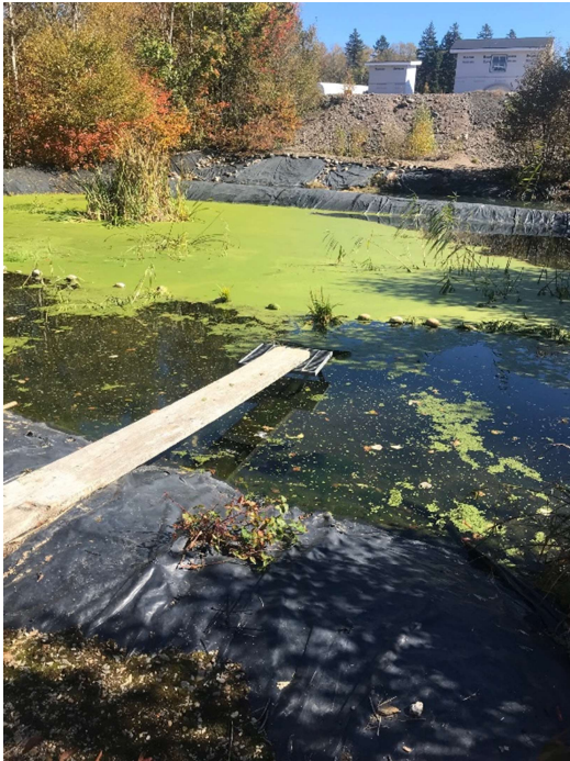
Photo 8 Existing Settling Ponds
