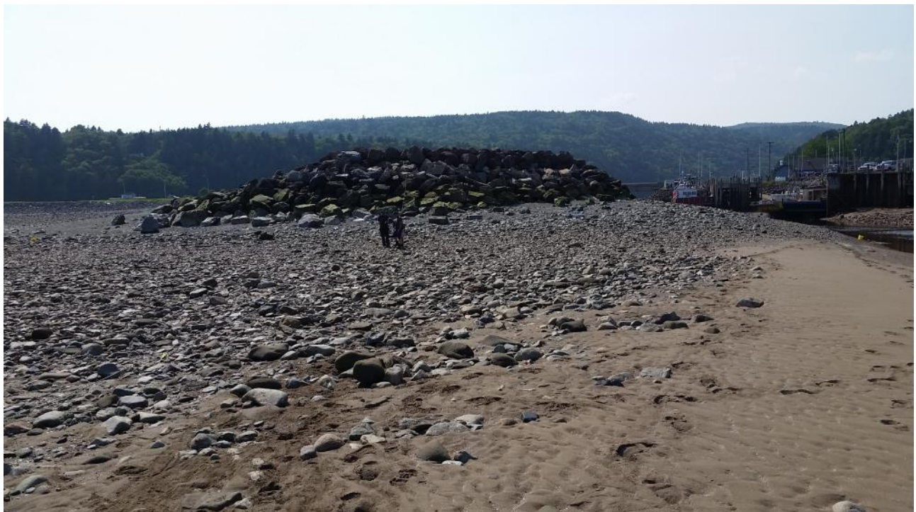
Photo from T2 B looking west towards existing breakwater
