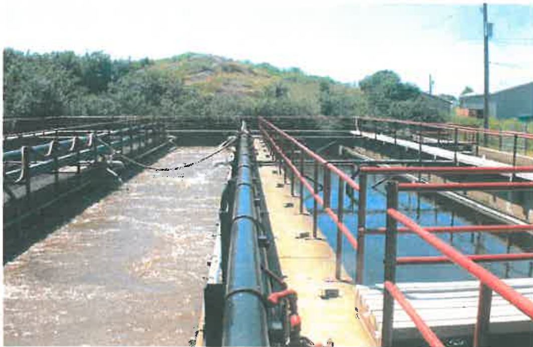
Figure 2 Looking west toward across the treatment lagoon.
