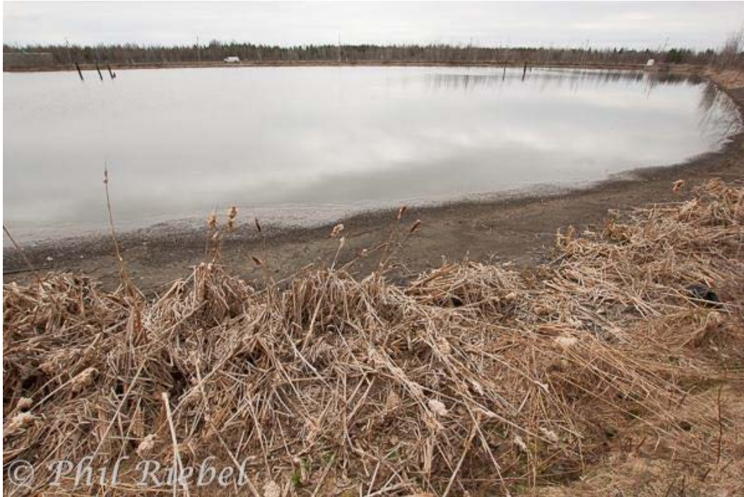
Figure 7-2a Vegetation Growing on Area of Exposed Sediment Along the Border of Cell No.3 of the ASB Looking Towards the Outfall Structure (Same area as Figure 7-2b but taken May, 2014)
