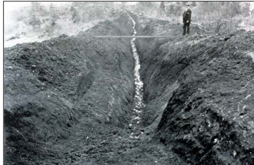
Draining water from a wad manganese deposit at Dawson Settlement, south-eastern New Brunswick, c. 1898. Bailey 1899
