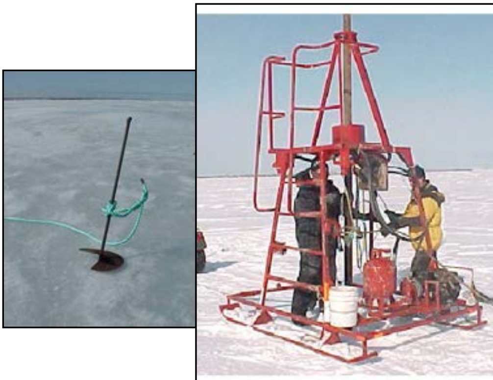
Figure 27 Helical screw anchor and hydraulic device
