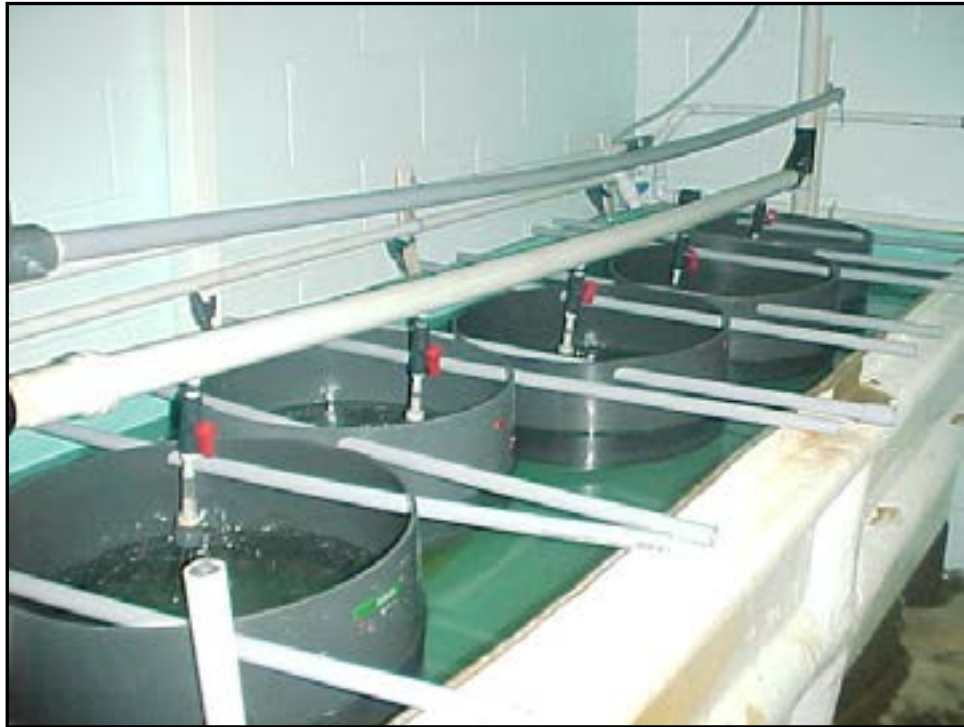
Figure 17 Downweller system used in hatcheries
