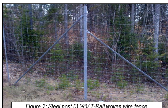
Figure 2: Steel post (3 1/2") T-Rail woven wire fence
