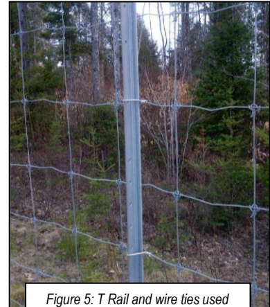
Figure 5: T Rail and wire ties used to hold woven wire against the T rails
