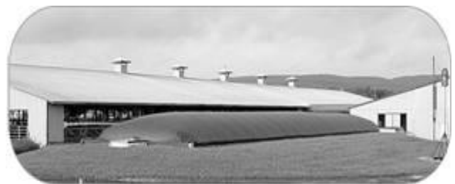
Fig 5. Plug flow anaerobic digester (Source: OMAFRA)
