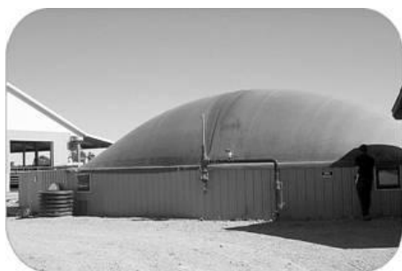
Fig 4. Completely mixed anaerobic digester (Source: OMAFRA)
