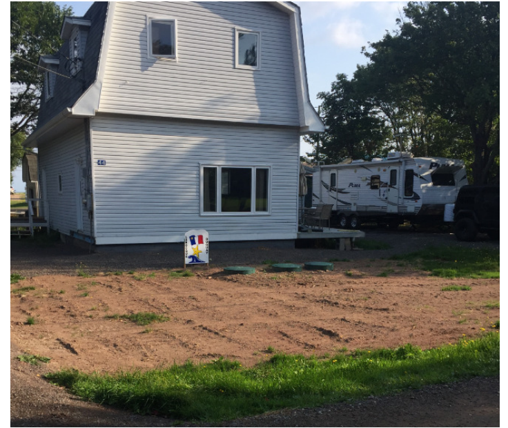
Newly installed septic system in Area 1C
