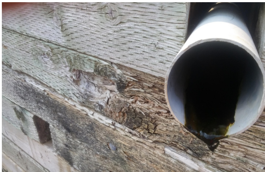
Drain pipe at beach, retaining wall in Area 2B
