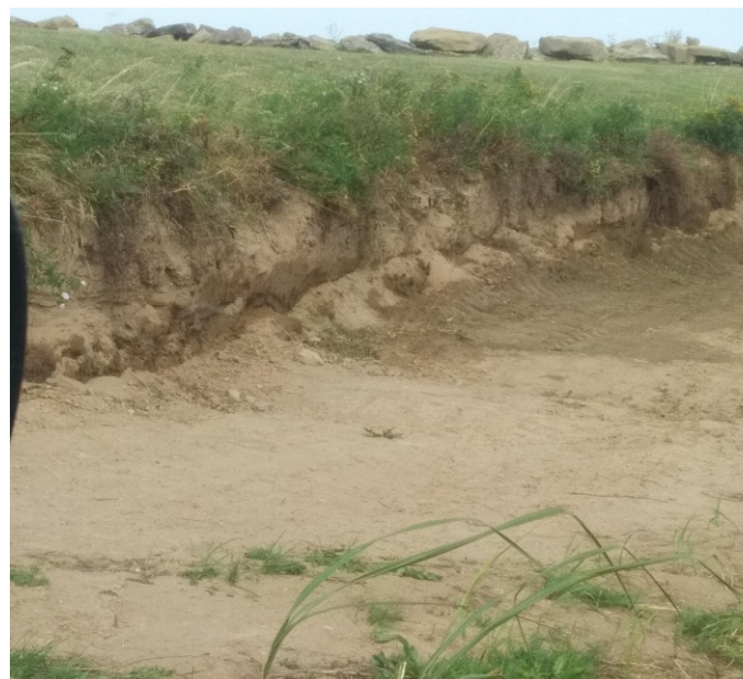
Excavation near beach in Area 1A
