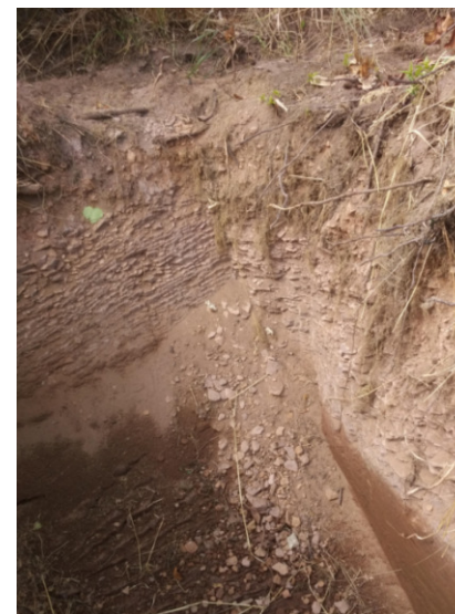
Test pit for new septic system in Area 1A
